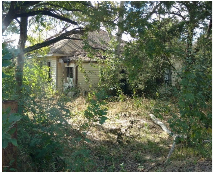
Figure 3B: Overgrown Yard/Dilapidated Housing Example
