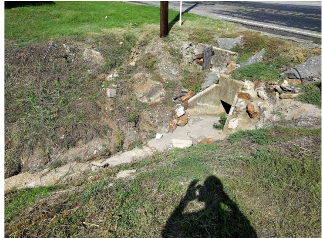
Figure 7B: Roadside Ditch Example
