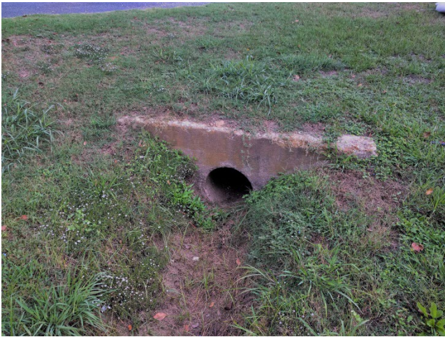
Figure 7A: Roadside Ditch & Concrete Culvert Example
