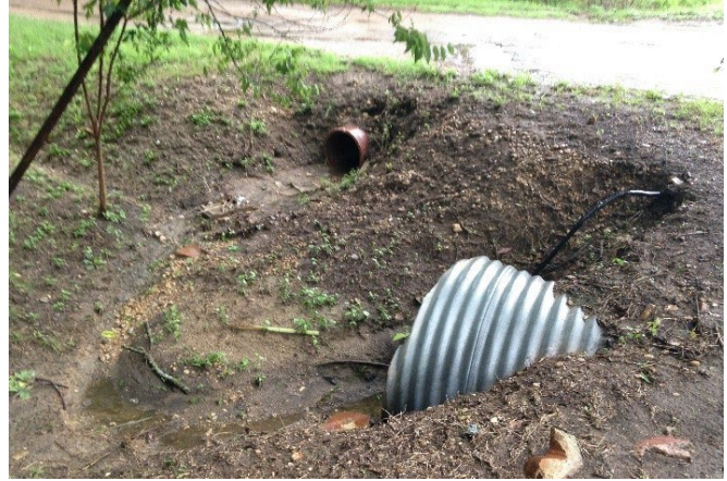
Figure 7D: Undamaged Culvert Example
